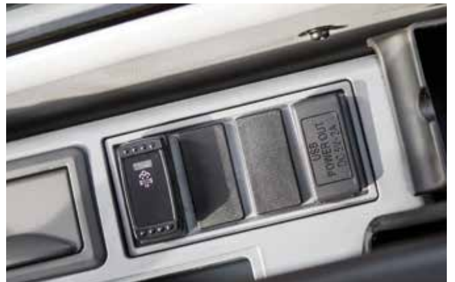
The USB power outlet is useful for charging portable devices such as mobile phones.
